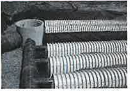
24" (600 mm) inlets are the maximum size that can fit into a SC-740/DC-780 end cap and must be prefabricated with a 24" (600 mm) pipe stub. SC-310 chambers with a 12" (300 mm) inlet pipe must use a prefabricated end cap with a 12" (300 mm) pipe stub.
