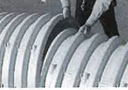
Continue installing chambers by overlapping chamber end corrugations. Chamber joints are labeled "Lower Joint - Overlap Here" and "Build this direction - Upper Joint". Be sure that the chamber placement does not exceed the reach of the construction equipment used to place the stone. Maintain minimum 6" (150 mm) spacing between rows.
