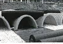
Place two continuous layers of ADS Woven fabric between the foundation stone and the isolator row chambers, making sure the fabric lays flat and extends the entire width of the chamber face. Drape a strip of ADS non-woven geotextile over the row of chambers (not required over DC-780). This is the same type of non-woven geotextile used as a separation layer around the angular stone of the StormTech system.
