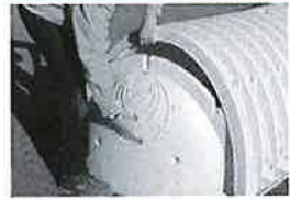
Lift the end of the chamber a few inches off the ground. With the curved face of the end cap facing outward, place the end cap into the chamber's end corrugation.
